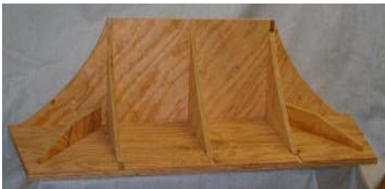
Plywood Soffit Canopy Support
